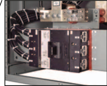
Fig. 13: Ground and neutral disconnect links
