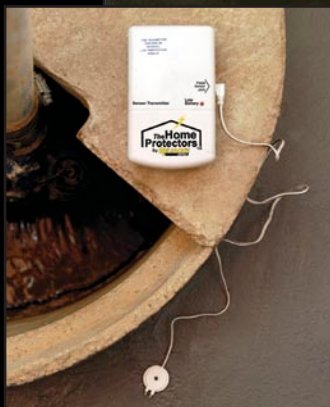
Transmitter shown near sump pump
